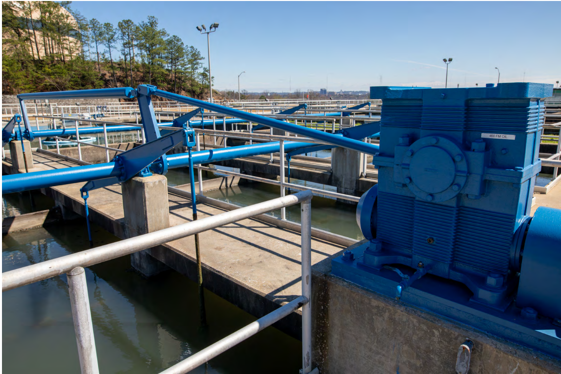
WESTERN FILTER PLANT
