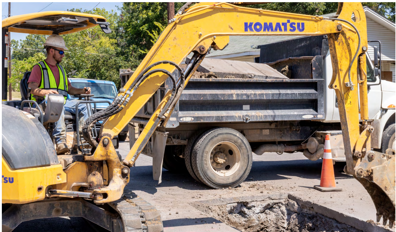
BWW CREWS WORK TO REPLACE PIPE AND PATCH THE ROADWAY
