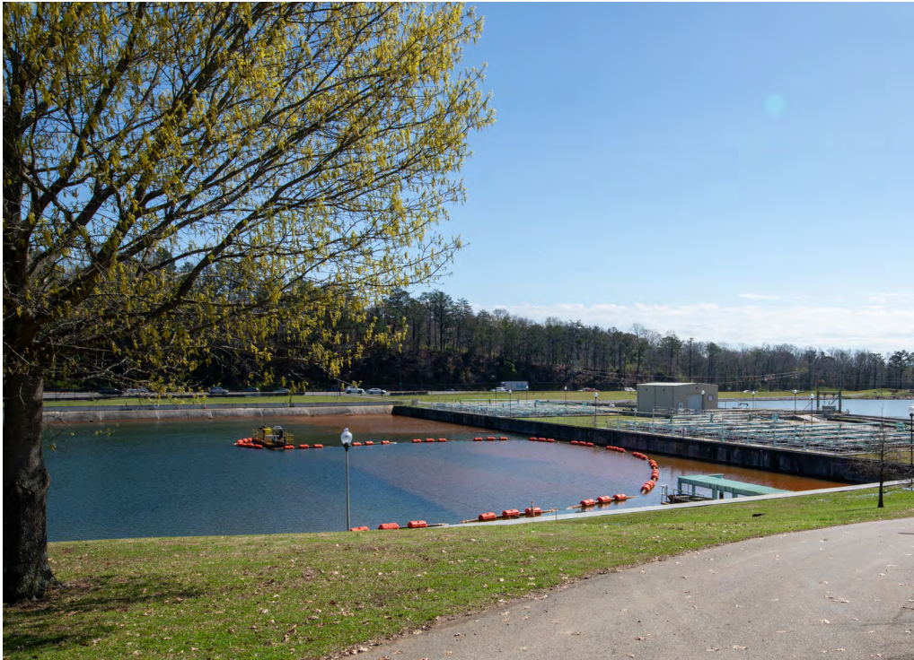
SHADES MOUNTAIN FILTER PLANT
