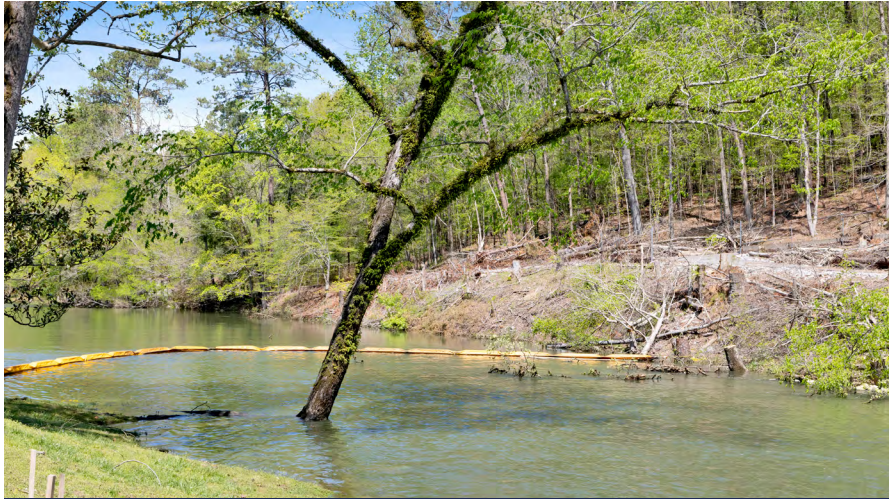
LAKE PURDY DAM CONSTRUCTION
