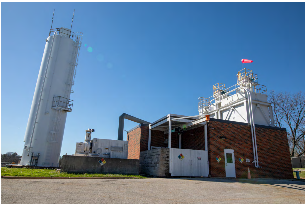
PUTNAM FILTER PLANT
